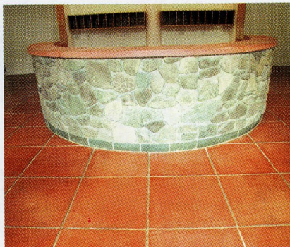
The finished colored slab in the new building is grouted in the trowel lines to create the effect of terracotta tiles.
