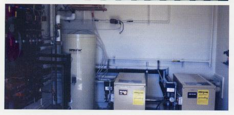
radiant boiler and provides partial boiler reset. The 252 controller also activates a high temperature zone from the high temperature boiler when the radiant boiler is unable to meet the load. Hot water is injected from the high temperature secondary loop into the return line of the radiant boiler.
