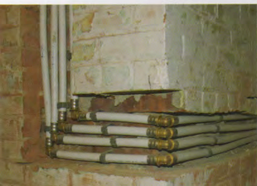
Bricks were removed from the chimney to conceal piping, then were cut down and set back in as a veneer.
