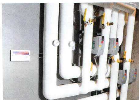
Wilo Stratos ECM pumps handle distribution for the radiant heat and air handlers for both heating and cooling.
