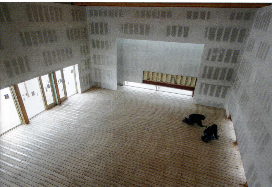
Abularrage's team worked tirelessly to put the radiant underlayment system in place.
